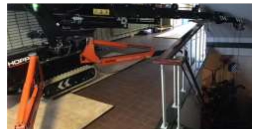
SET IN CONFINED SPACE
